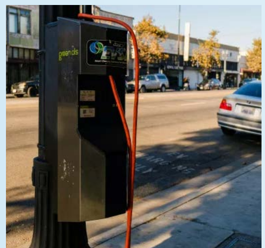
Street light outfitted with electric vehicle charging infrastructure in Los Angeles. Credit: Electrek
